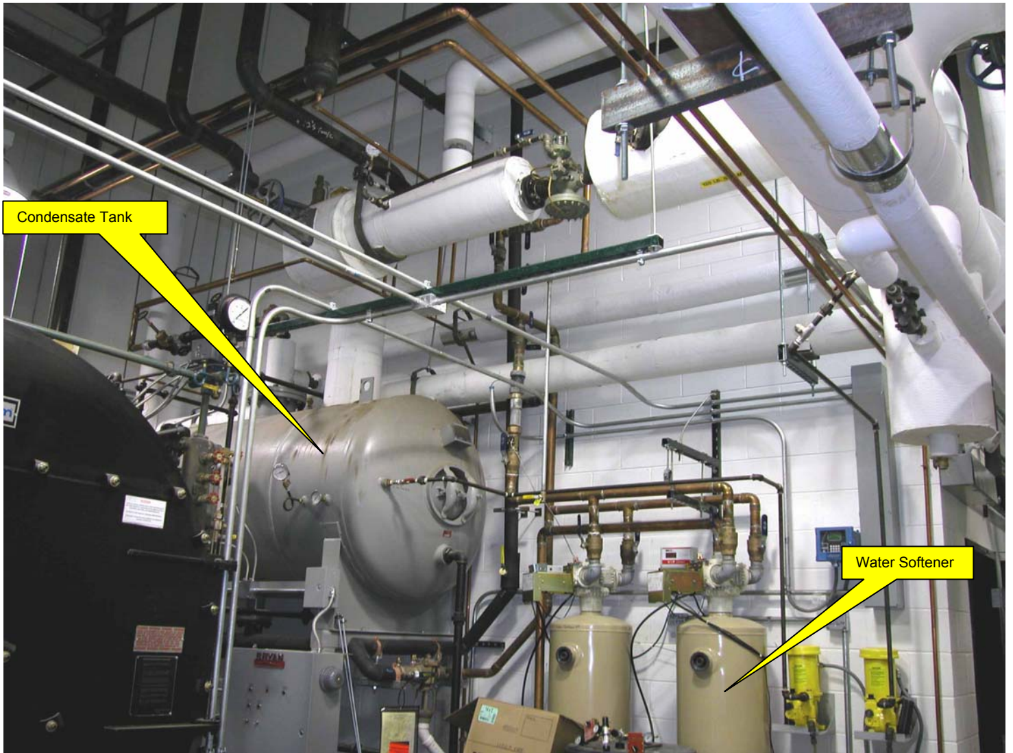
Figure 11 Condensate System
